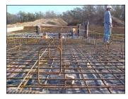
The rebar and added mesh is what keeps the concrete from splitting apart. It is the actual strength of the foundation.
